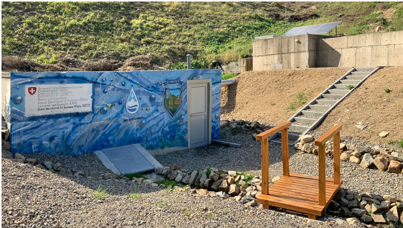
Rehabilitated intake structure below Loshana dam
