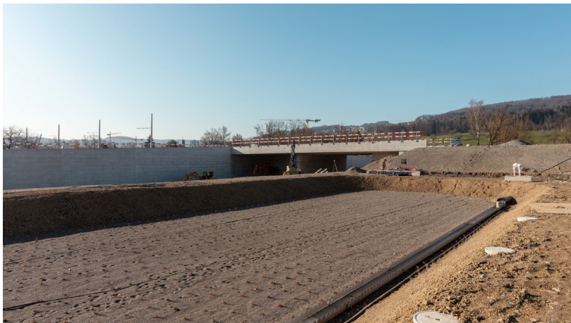
Treatment facility for road runoff at the Mutschellen junction. Picture Credits: © bürobureau
