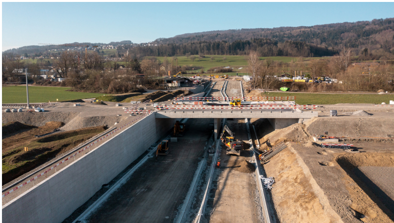
Mutschellenstrasse with new overpass. Picture Credits: © bürobureau
