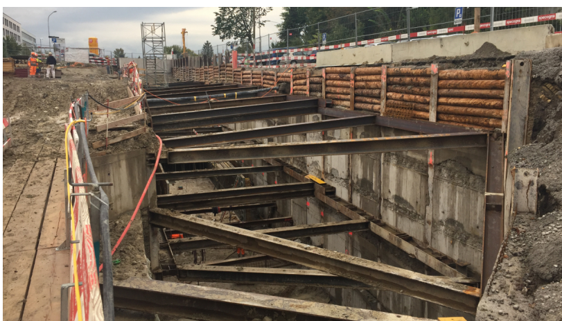
Construction pit for tunnel link
