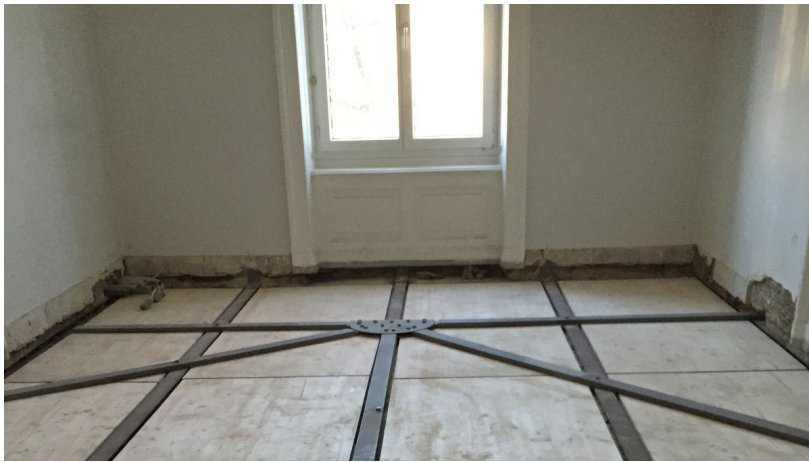
Ceiling structures (Picture Credits: EBP)
