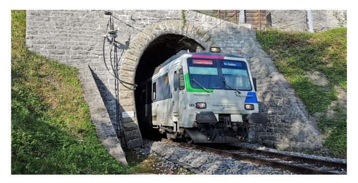
Swiss Southeastern Railway has commissioned EBP to complete the planning for the necessary renovation of the Sturzenegg Tunnel, which was originally built in 1910. The aim of the renovation measures is to guarantee compliance with the applicable structure-gauge requirements and to secure the tunnel's serviceability and long-term structural integrity. The scope of EBP's work also includes issuing invitations to tender and managing the project's realization.
