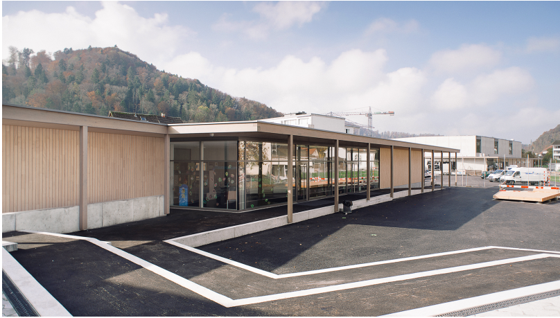
School building and connecting corridor
