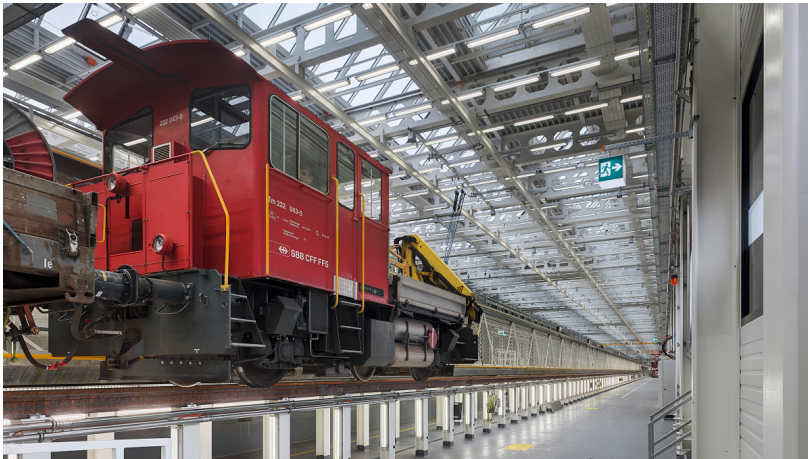
Serviceanlage Herdern innen
